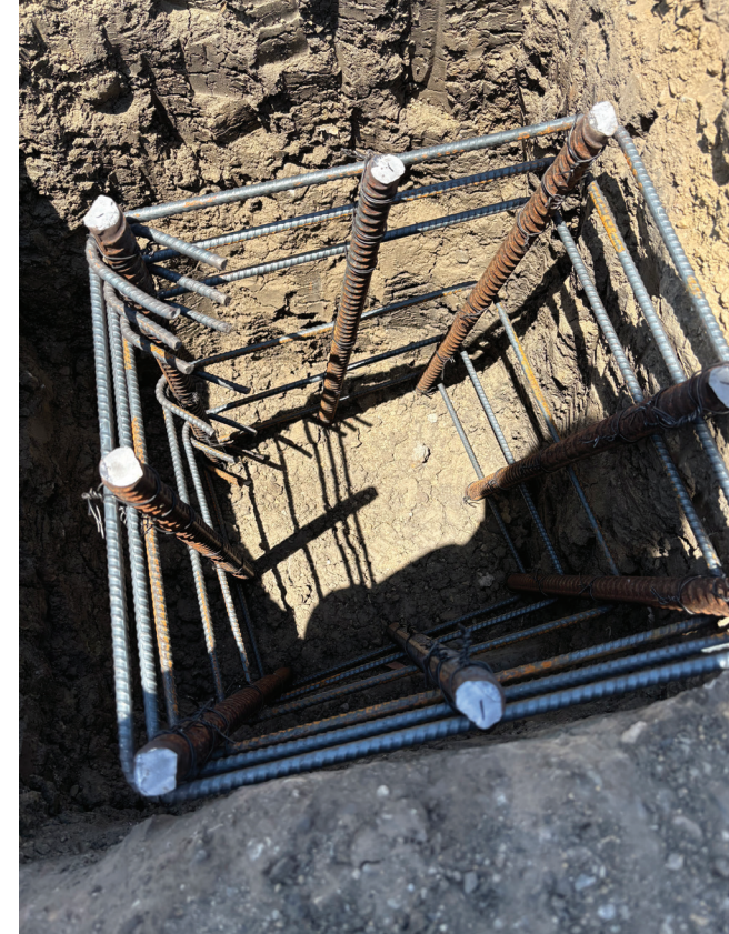
⌚ Rebar reinforcement and forms in place, ready for concrete pour; completed footings provide a solid foundation for the pergola.
