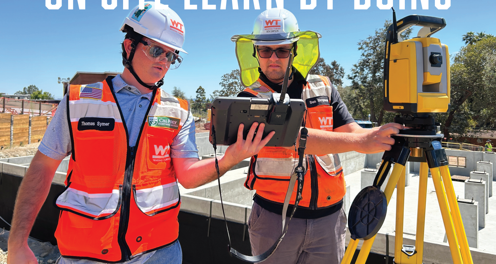
Ⓢ Thomas Symer (CE, student, left) and Ben Simpson (CE, '24, right) set up Whiting-Turner survey equipment to verify anchor-bolt locations to within 1/8"
