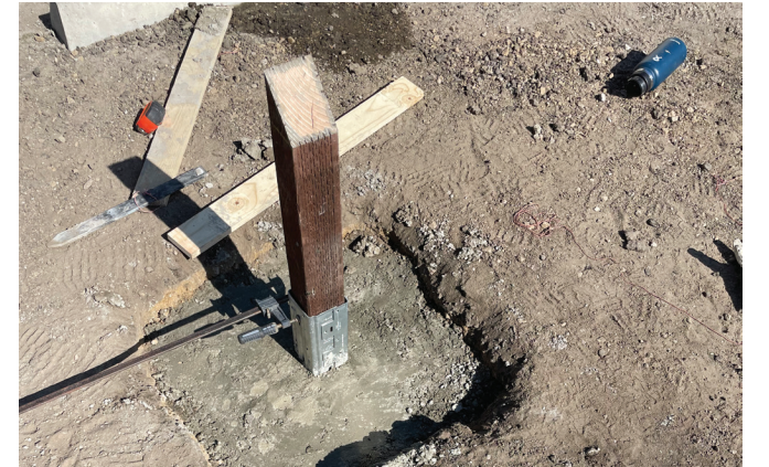
⌚ Students work on framing the pergola, installing columns and Simpson Strong-Tie connections during their senior project build.
